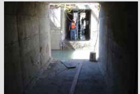
Ensenada International Terminal Tunnel, Mexico
