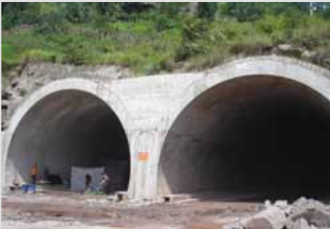
Yunnan Shuima Tunnels, China
