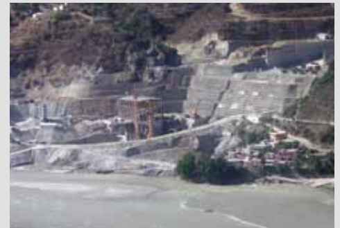
Alakanada Dam, India
