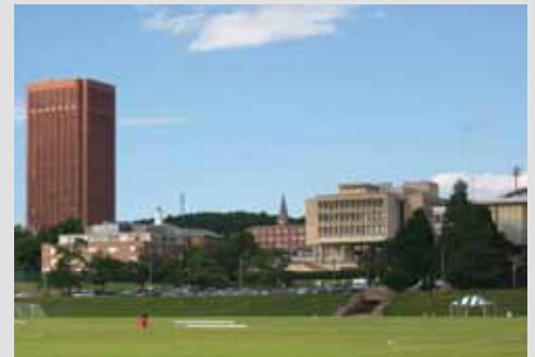
UMass Amherst - Boyden Tunnel, USA
