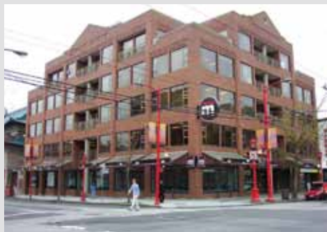
Channel M Building, Vancouver, Canada
