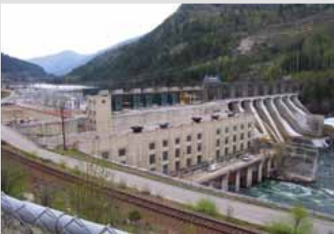
BC Hydro's Bridge River Complex, Canada
